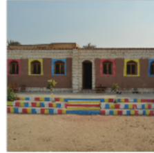
Behbeit school (Painting walls)
