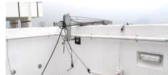
Strengthened Parapets to fix gondola
