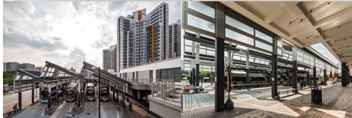
Upon completion, noise performance was verified by on-site measurement and the result was satisfactory
