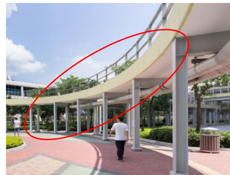
Provide railing to all roof
