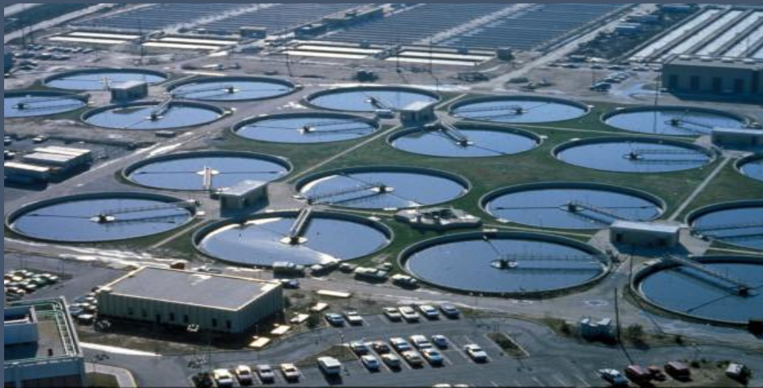
Nicosia Waste Water Treatment Plant
